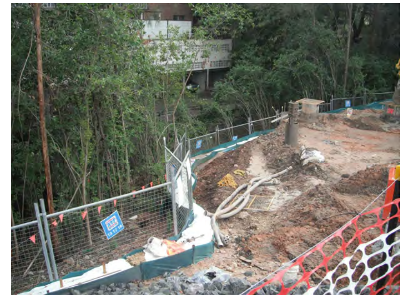
PHOTO 2: MODULAR SEDIMENT TRAP EXAMPLE
