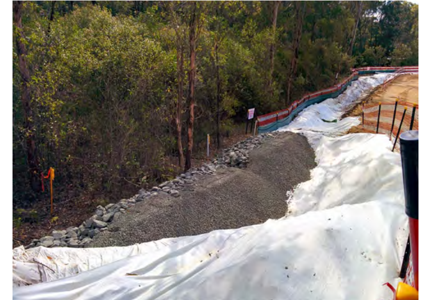
PHOTO 1: ROCK FILTER DAM EXAMPLE
