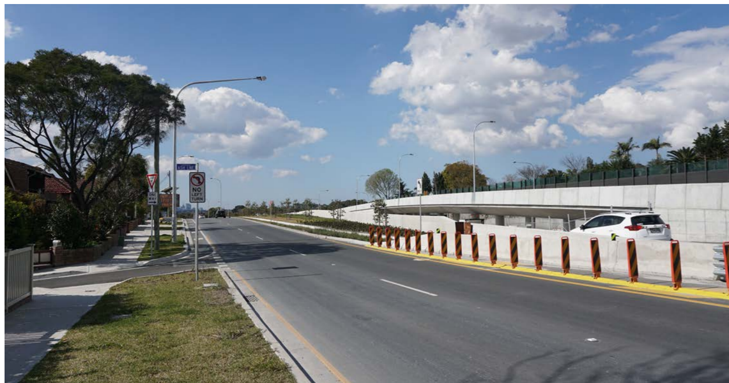
Figure 3-19: View along Wattle Street looking towards entry portal
