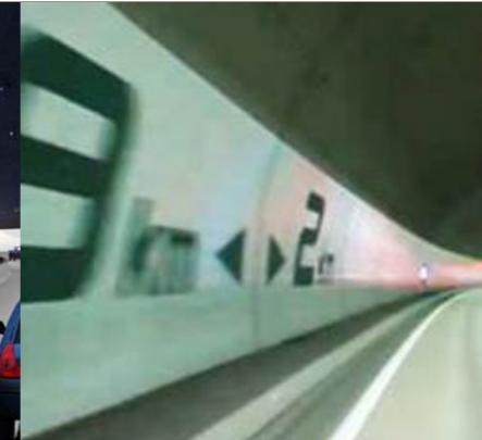
Hida tunnel, Japan
