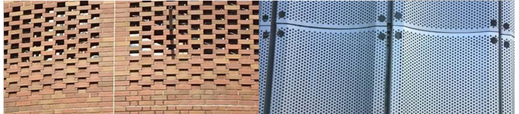
M4 East, Parramatta Road Ventilation Facility
