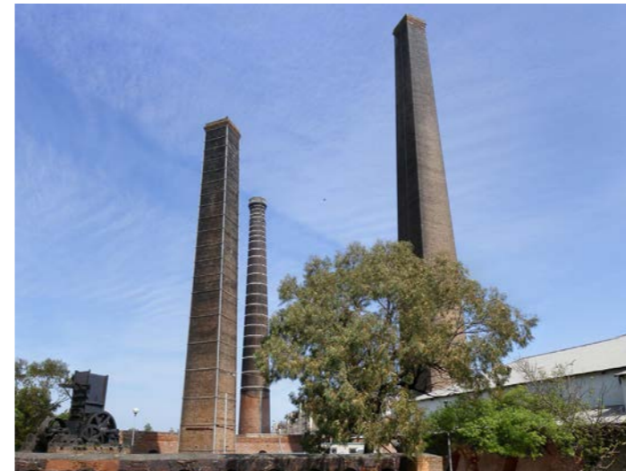
Figure 3-24: Existing brick kilns
