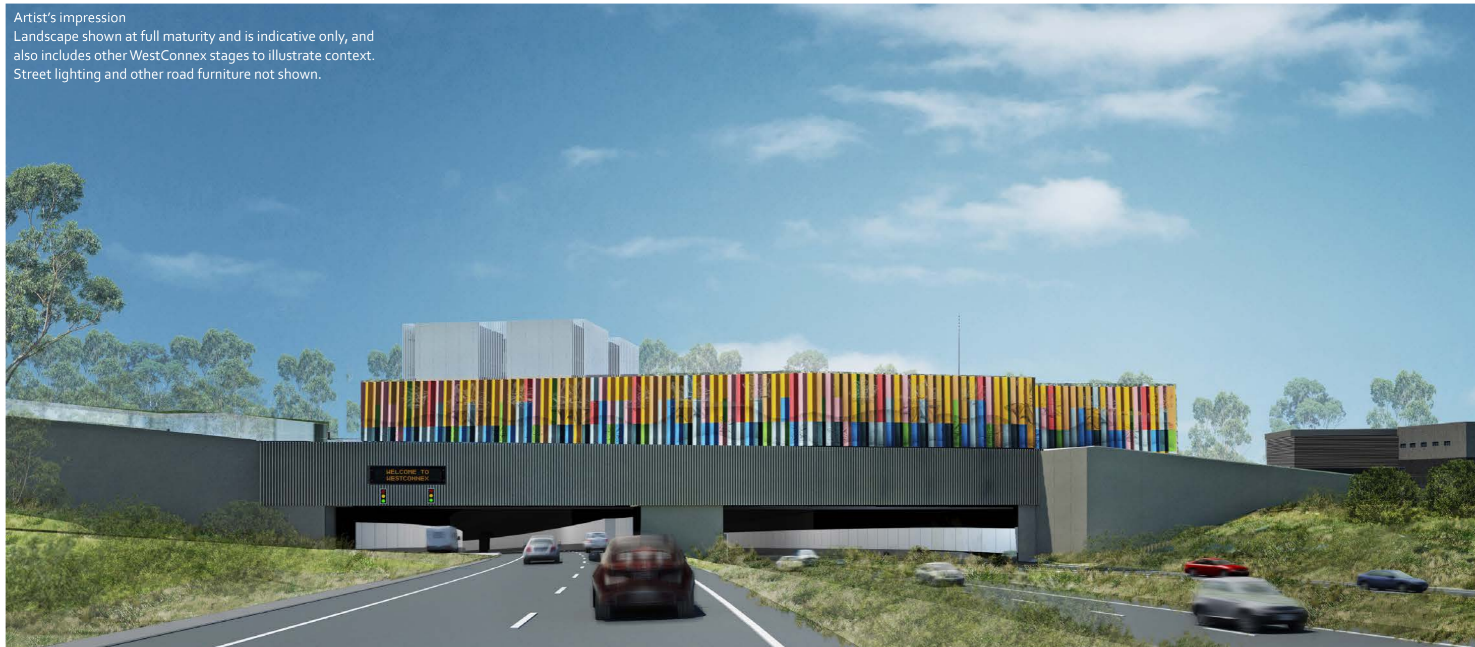
Figure 5-40: Campbell Road ventilation facility – view looking north
