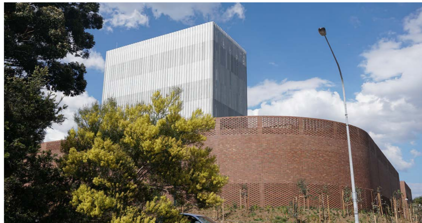
Figure 3-20: View of Parramatta Road ventilation facility
