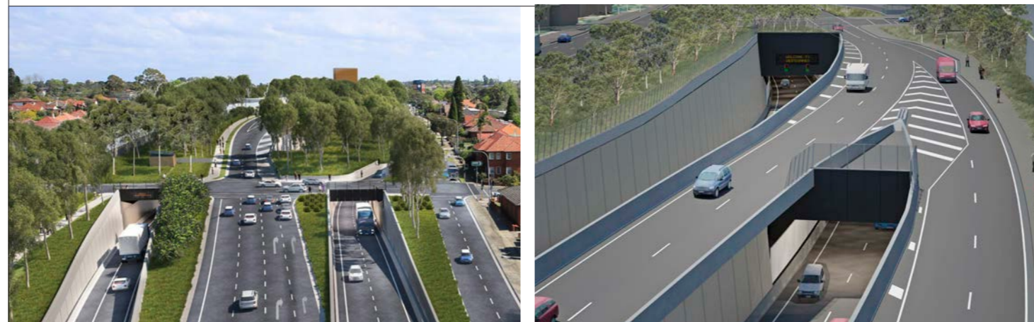
M4 East - Portal dive structure at WSI
