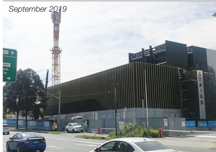
New M5 - St Peters MOC 4 (view from Canal Road)
