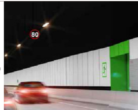
M4 East tunnel
