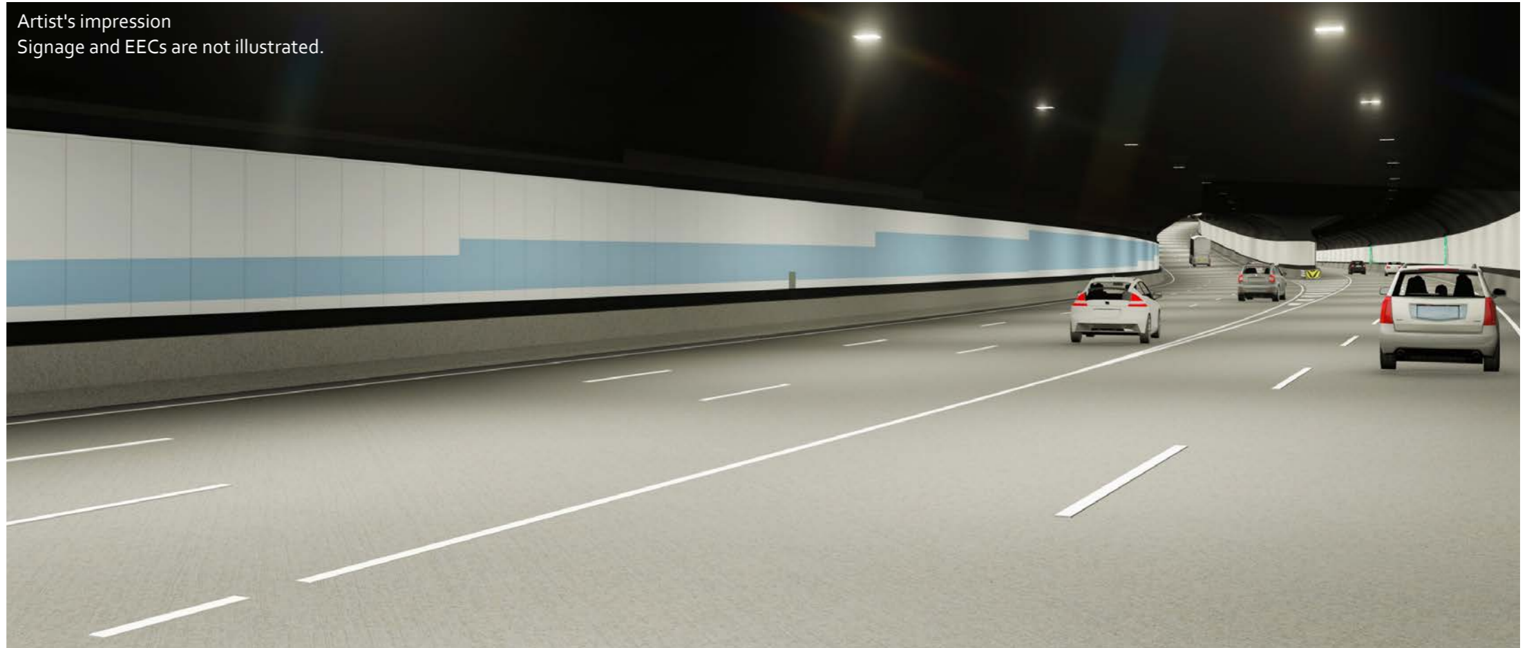
Figure 6-10: Tunnel exit marker (exit ramp to M4-M5 Link Rozelle interchange shown in its final configuration)
