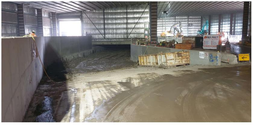
Photo 7: Backfilling tunnel ramp
