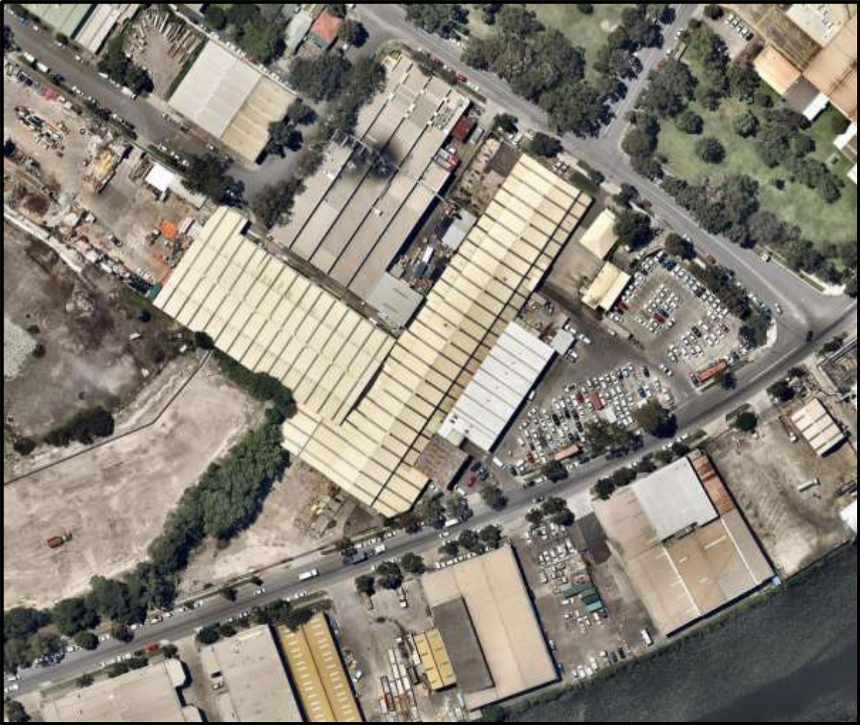
Figure 2. Aerial view of subject property (Source: Nearmap, accessed 17.11.15).
