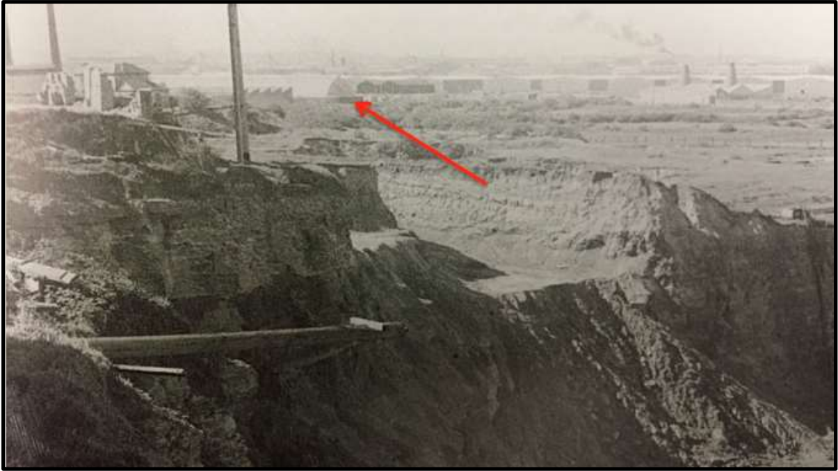
Figure 6. The Austral pit which was shared by The Central Brick & Tile Co Pty Ltd. The first building on the subject site can be seen in the background (indicated by red arrow).
