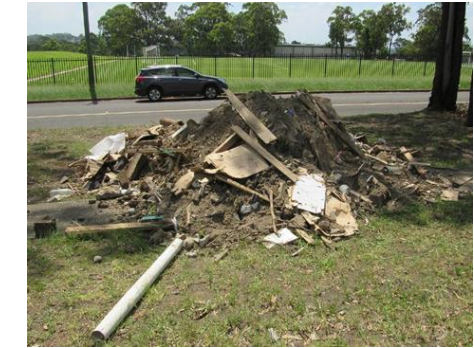
Figure 1 Excavated asbestos and building material
