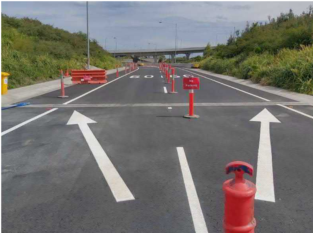
Figure 2-3 Permanent asphalt and line marking, St Peters October 2022
