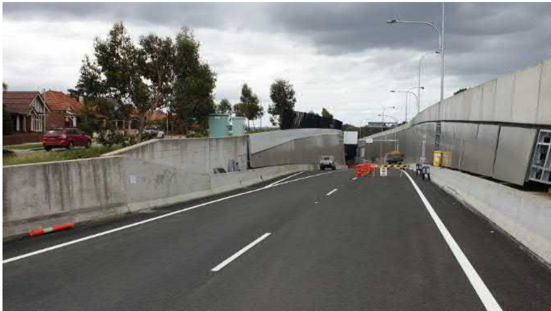
Figure 2-2 Wattle Street Cut and Cover works near to completion, March 2022
