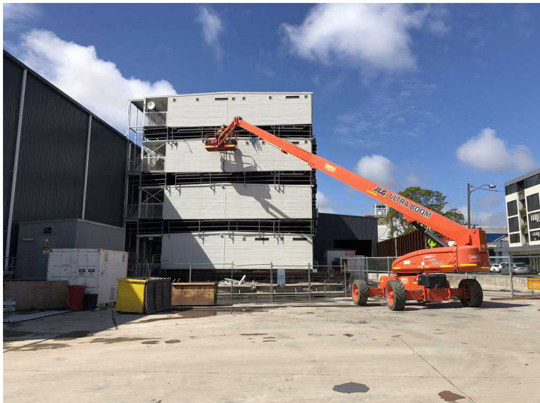
Figure 2-4 Pyrmont Bridge Road Office Removal October 2022
