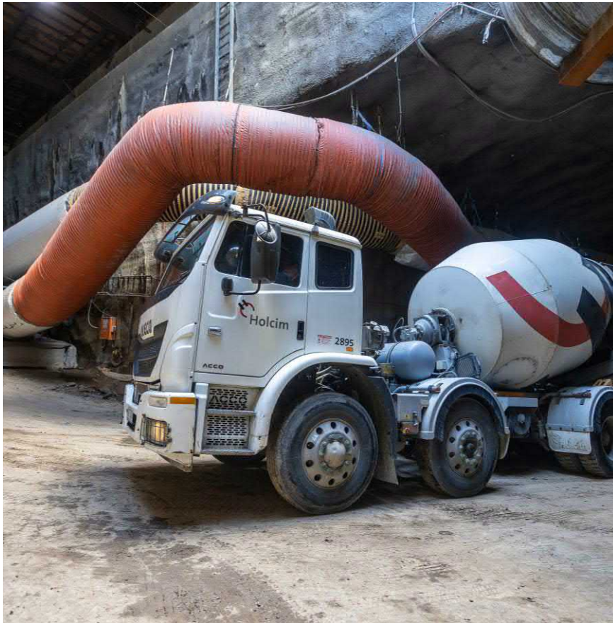
Figure 2-1 Adit backfill: flowable grout being poured, St Peters October 2022
