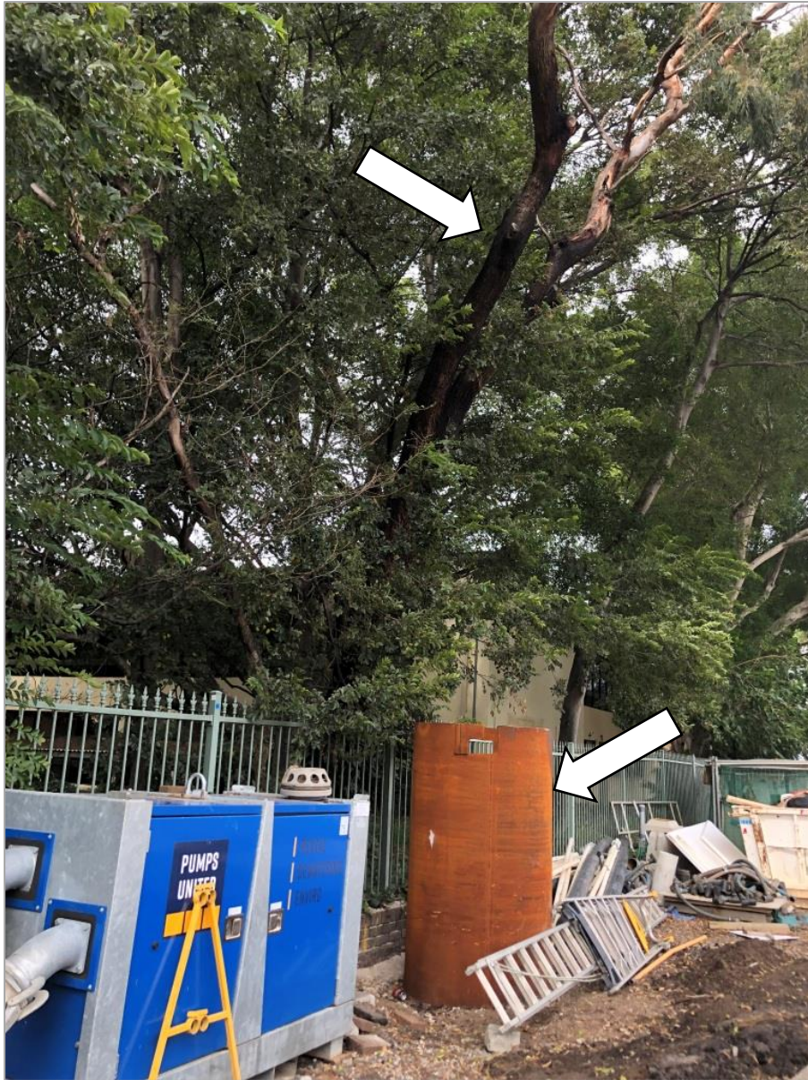
Plate 2 – Arrows note subject tree and VMS footing.
