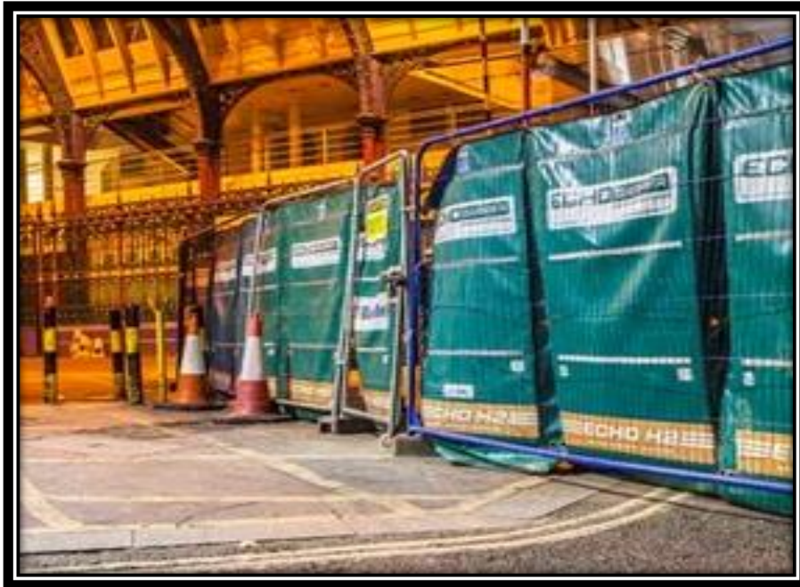
Figure 2: Temporary noise screens
