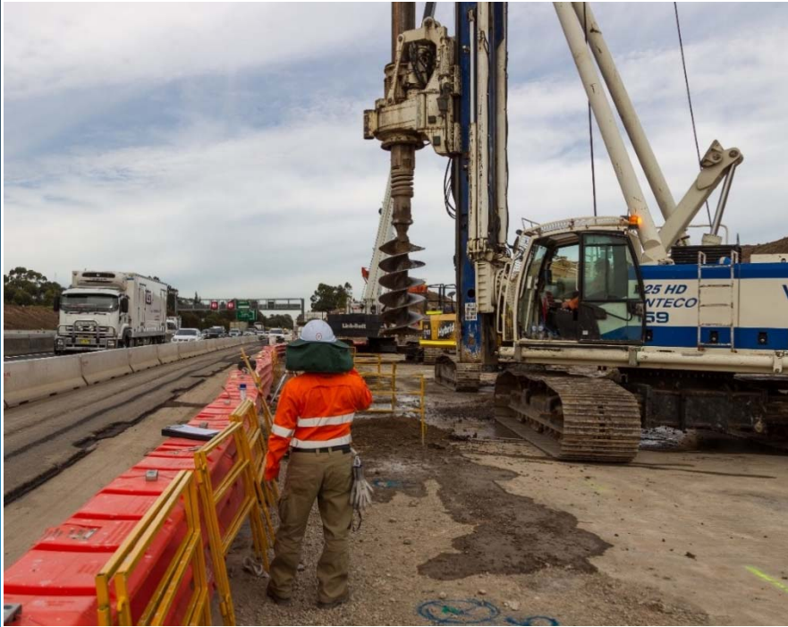
Bored piling off the M5 East Motorway, Oct 16
