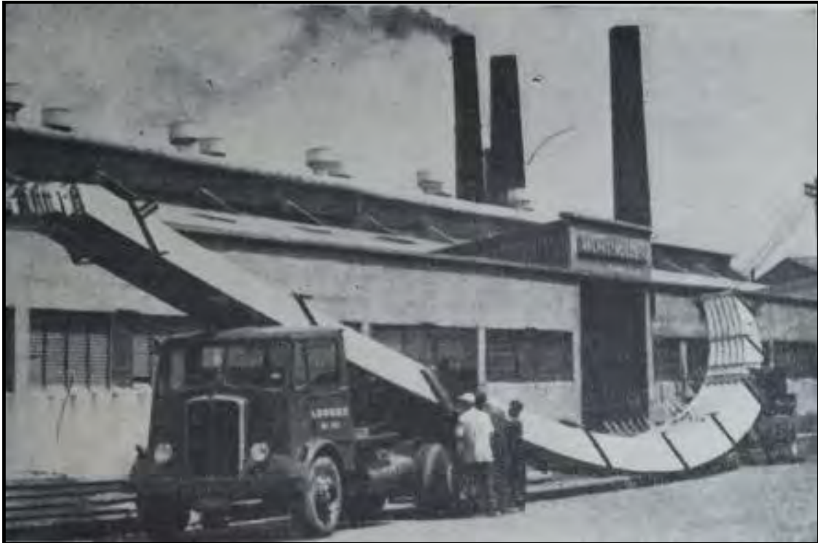
Figure 33. Laminated timber arches manufactured by Ralph Symonds Ltd, Sydney, for transportation to Melbourne for the Neon Industries building (Source: “120ft Laminated Timber Arches, Transported from Sydney to Melbourne. Building Lighting Engineering, 24 March 1955 p.33. NSW State Library).
