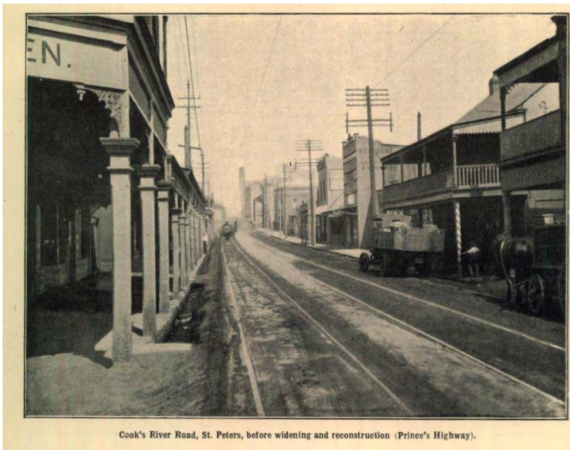
Figure 5. Cooks River Road (now Princes Highway) in St Peters showing former buildings and tramway, circa 1925, view from Campbell Street looking south (Source: Main Roads Board of NSW First Annual Report 1925-26 p.9).
