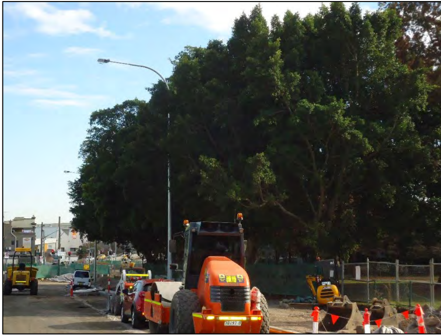
Photo 3: Light pole 80 adjacent tree 148.
