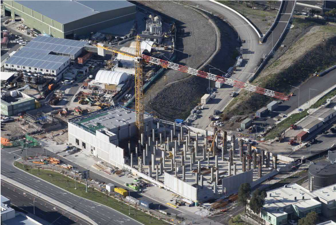
Figure 2-3 - Aerial view of the ventilation building at the Campbell Road site in March 2021
