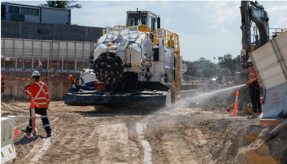
Image: the last roadheader for the Rozelle Interchange moving into the tunnel portal to start excavating from Iron Cove tomorrow.
