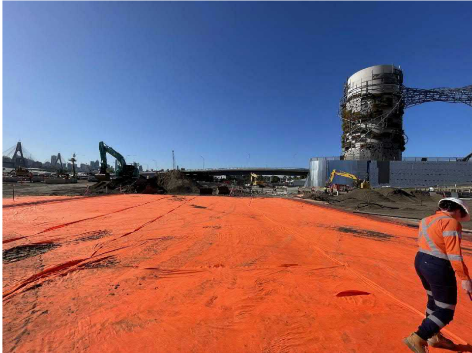
Figure 5.2 Geotextile marker layer
