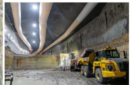
The below image shows inside a tunnel during benching, where work is carried out to remove the tunnel floor
