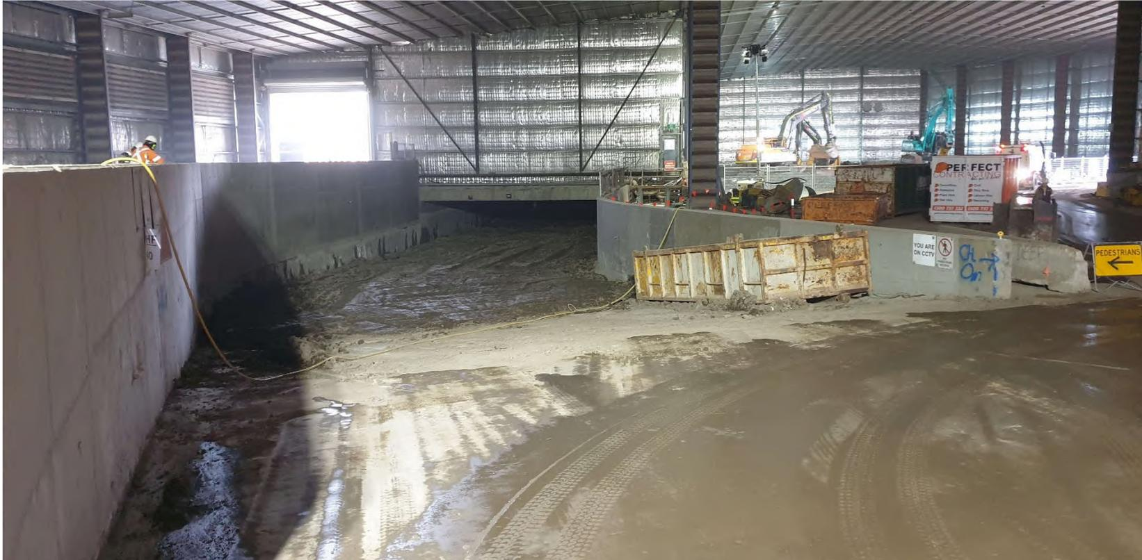
Photo 7: Backfilling tunnel ramp
