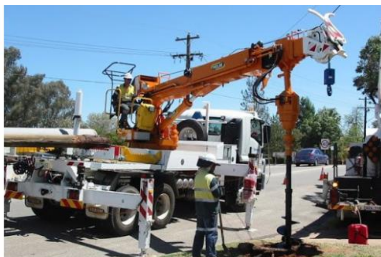
Image: Boring drill typically used during excavation and pole installation work
