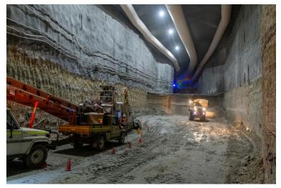
This image shows inside one of the substation caverns while we're 'benching'. Benching refers to the removal of the bottom part of the tunnel, or the tunnel floor, seen in the distance.
