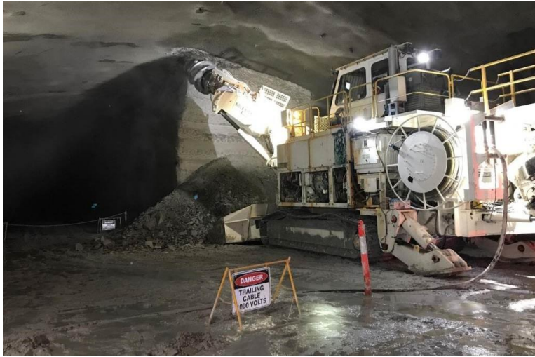
A roadheader inside one of our traffic tunnels. The roadheader cuts the rock using a rotating head on a moving boom as shown in the image
