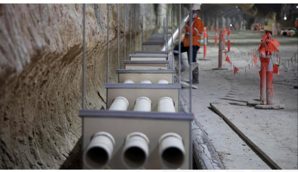
• In-tunnel civil work – around 4% of tunnel has final road surface
