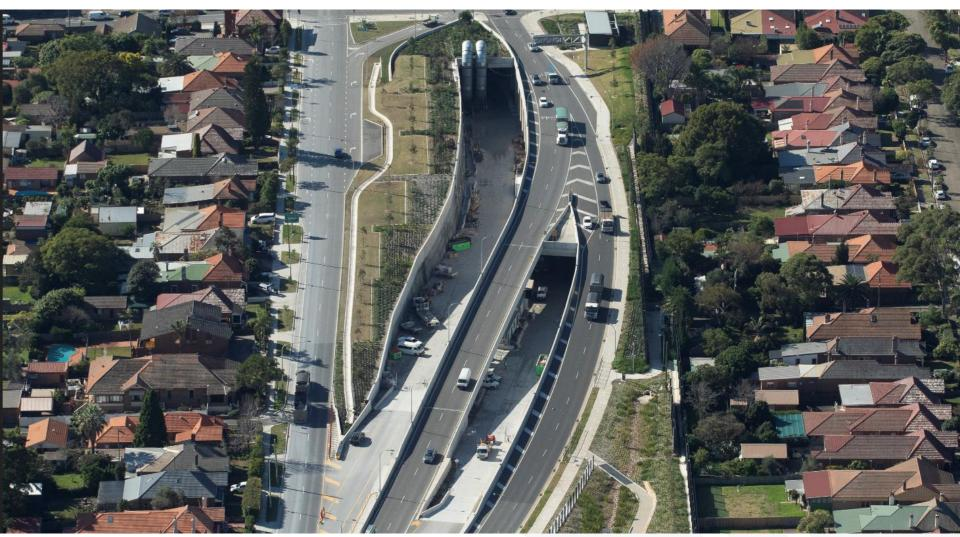
• Sandstone from the tunnel used for subgrade layer
