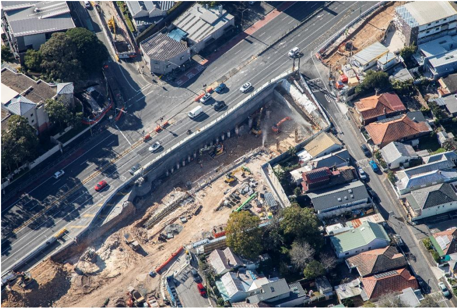
The 'cut-and-cover' on Victoria Road between Toelle and Callan streets
