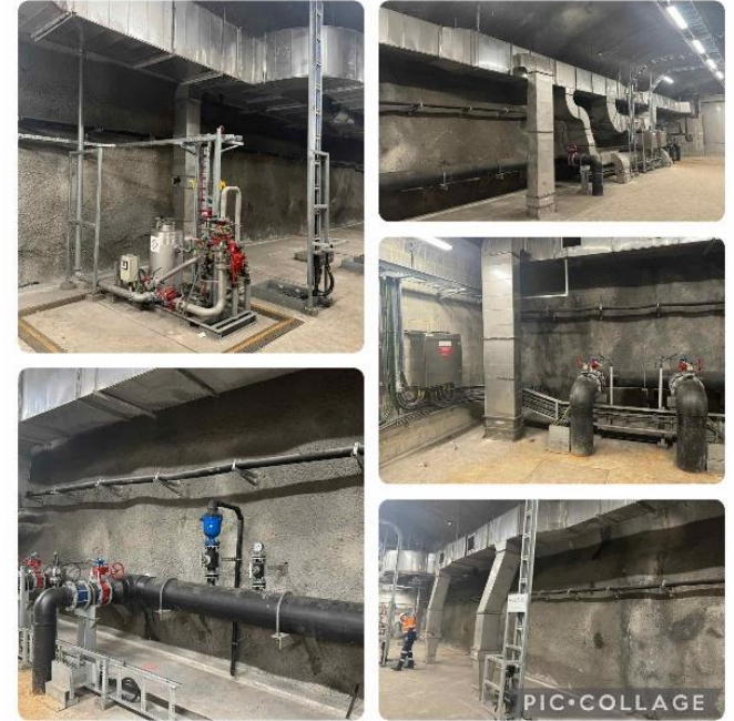
Building Structural Inspections
