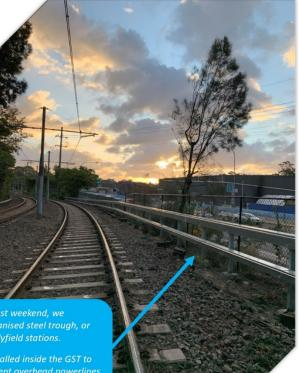
installed the last section of galvanised steel trough, or GST, between Rozelle Bay and Lilyfield stations.
