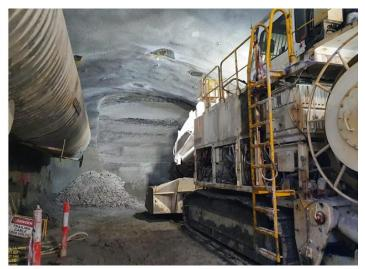
These images show roadheader tunnelling machines inside the new tunnels being excavated near the Rozelle Railyards. The majority of the Rozelle Interchange tunnels are excavated using a roadheader, which is a special excavation machine that cuts the rock in a circular motion.
