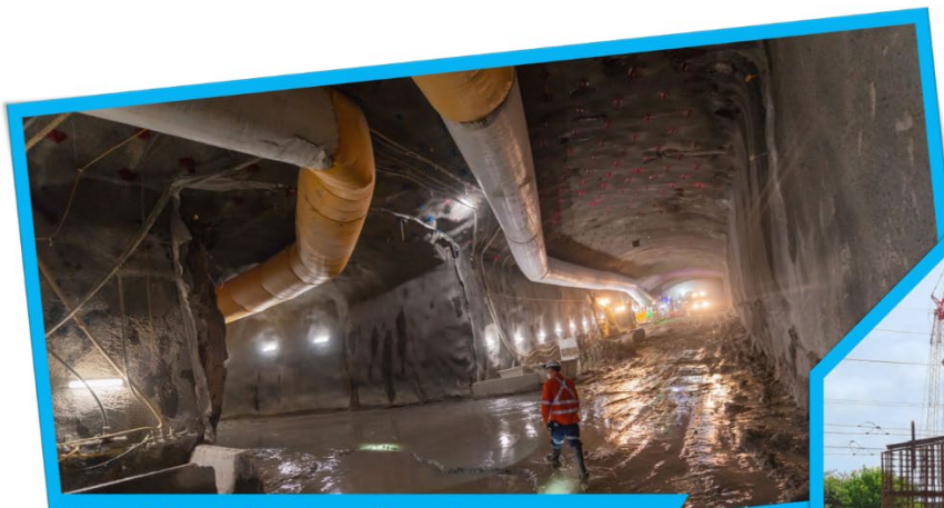
Inside one of the future Rozelle Interchange ventilation tunnels:
