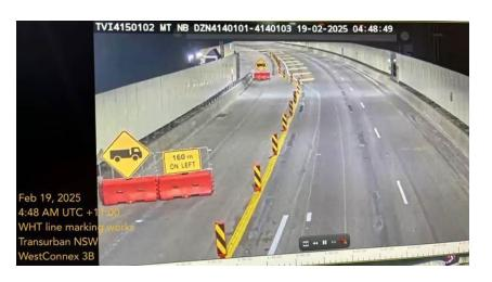
WCX has been working with TfNSW and the WHT D&C Contractor to complete lane adjustments within the Rozelle Interchange allowing for construction vehicles to use the live tunnel directly which will significantly reduce the number of trucks each day on the surface roads above (est. 1000 per day to use tunnel instead)
