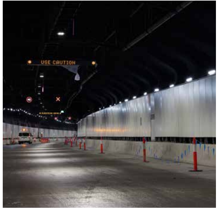
Lights on in the tunnel
