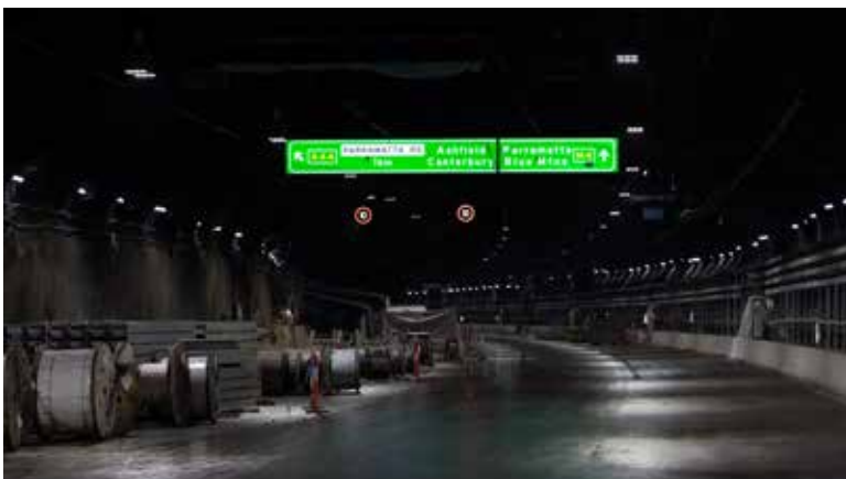
Newly paved road surface
