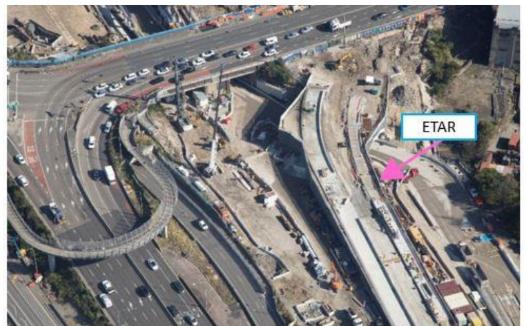
Image showing construction of the Eastern Temporary Access Road (ETAR) looking towards Victoria Road
