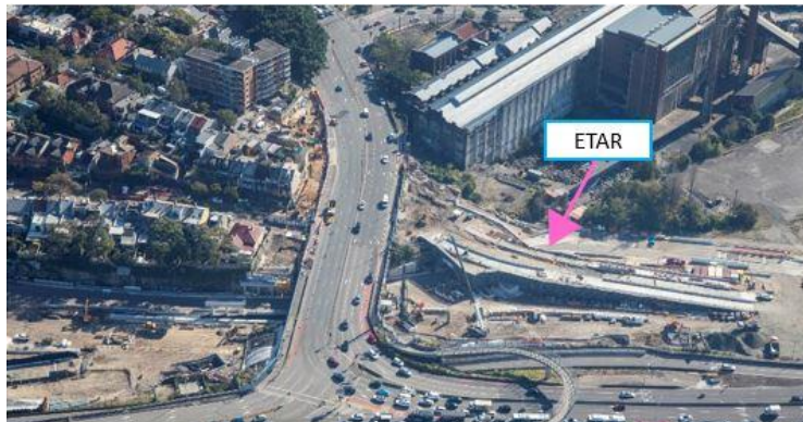
Image below shows the Eastern Temporary Access Road (ETAR) being constructed. This road will eventually be used by cars travelling from Victoria Road to ANZAC Bridge until the Victoria Road bridge is rebuilt.
