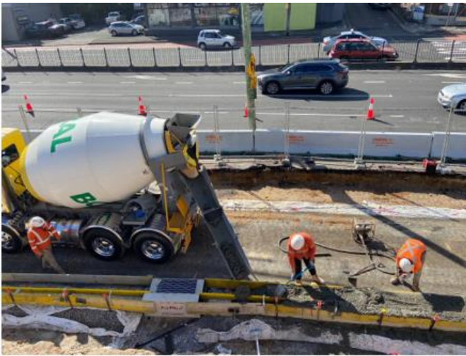
We are working to install a new kerb and gutter for the new Victoria Road traffic lanes between Springside and Callan streets
