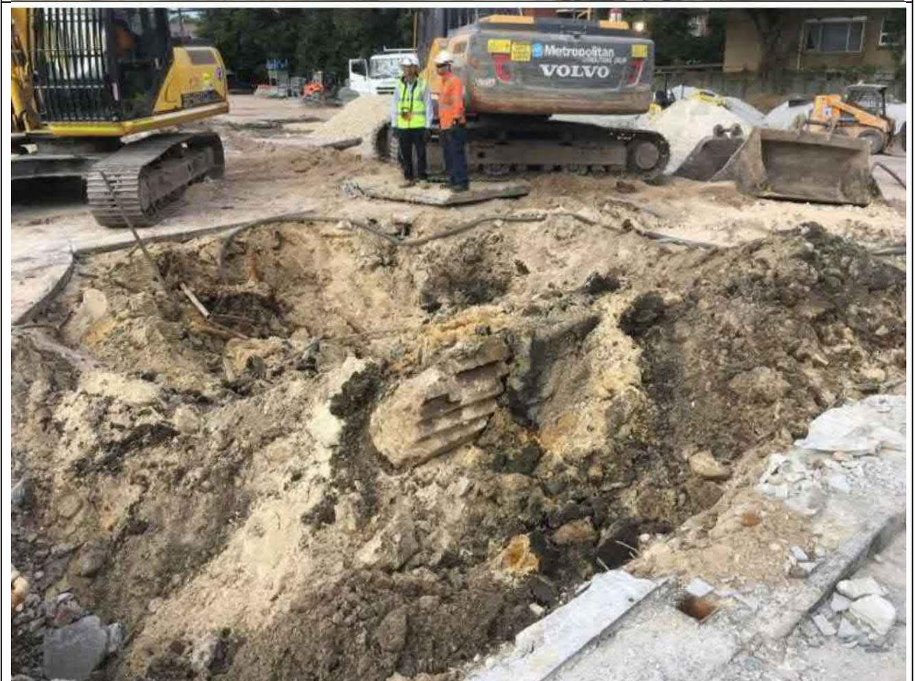
Figure 3-8 Photos of UST Removal at PREW site on 8/05/19 (Sheet 2 of 3)
