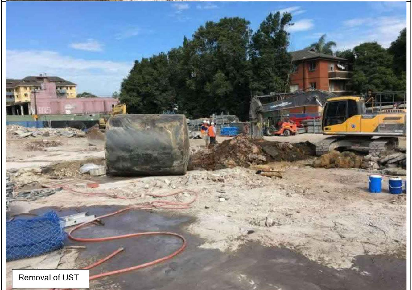
Figure 3-6 Photos of UST Removal Operation at PREW site on 2/05/19 (Sheet 2 of 2) (Source: Ref [5])
