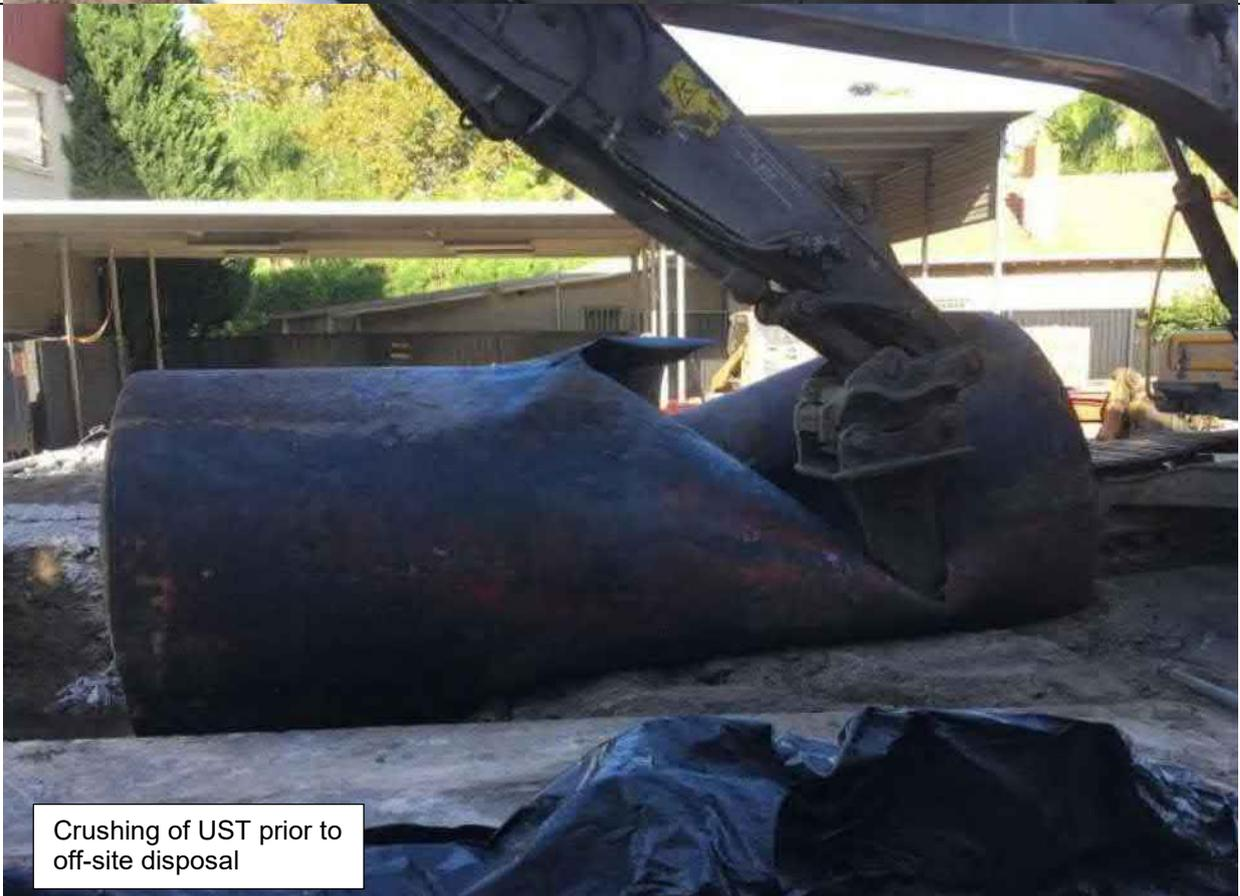
Figure 3-5 Photos of UST Removal Operation at PREW site on 26/03/19 (Sheet 2 of 2) (Source: Ref [5])
