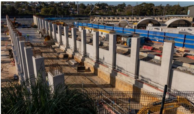
Picture shows the supporting foundations taking shape to the future entrance/exit of the M8 tunnels. The roof will be placed on top of these structures towards the end of the year.
