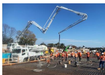
A concrete pump moves wet concrete from the agitator to the pre-installed steel framework
