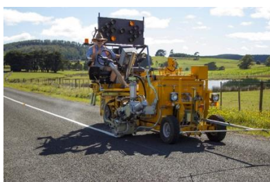
Line marking machines paint traffic signals on the new road
