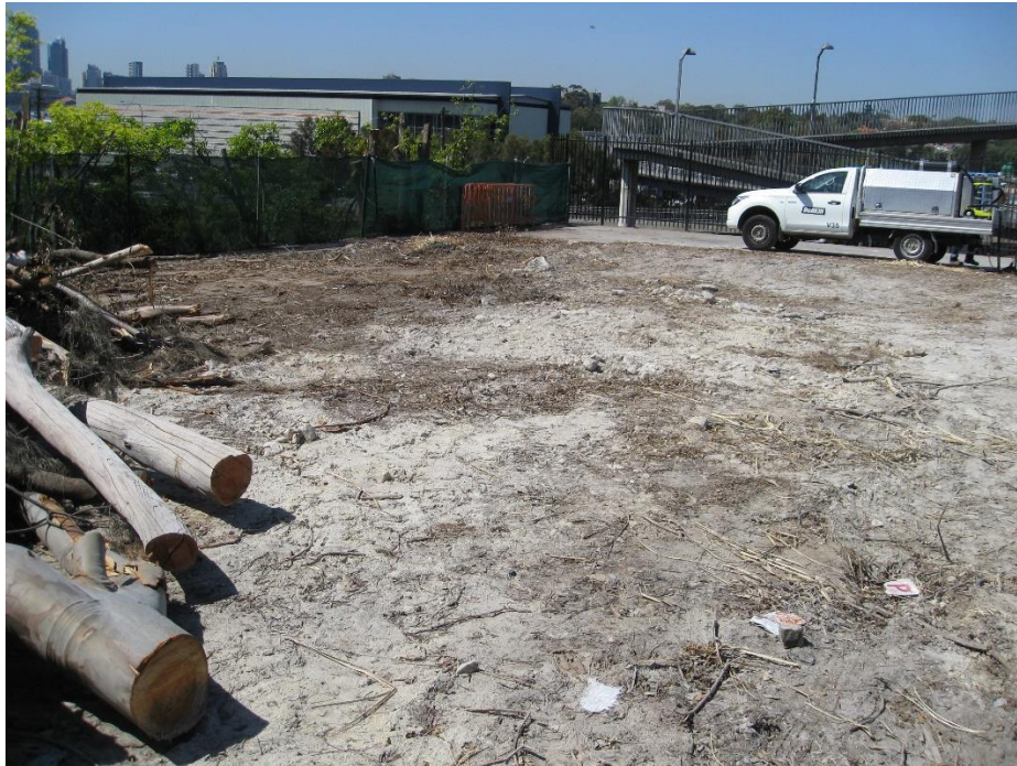
Figure 12 Site following removal of vegetation, looking southeast, October 2019 (Source: Extent Heritage)
