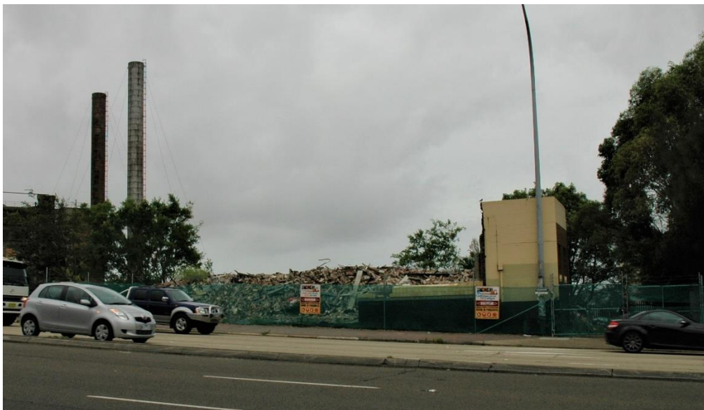
Figure 10 Remains of the hotel, April 2009. (Source AHMS)
