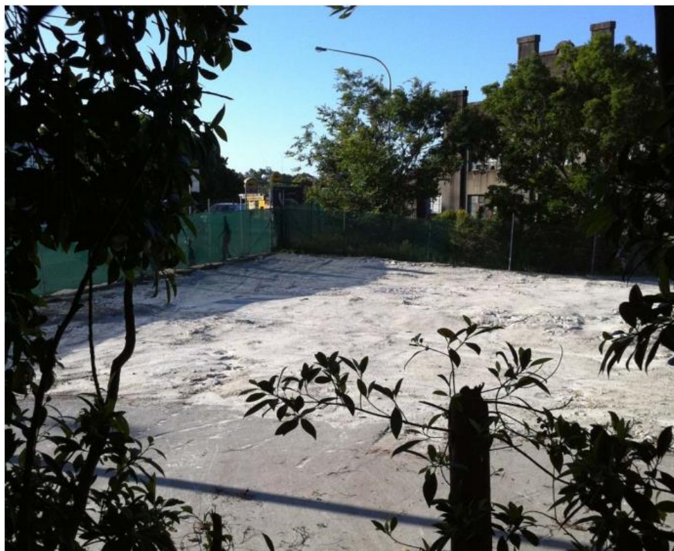
Figure 11 The site (looking north) following removal of demolition rubble and the laying of sand across the site, 2010 (Source: RTA 2010 p.23)
