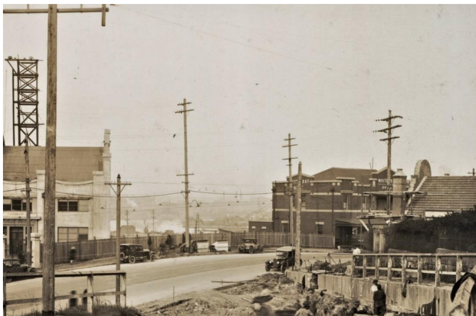
Figure 6 View of the White Bay Hotel (at right), 1926 (NSW SRA E5 - Weston Road, Balmain - Widening - Grading of side street NRS-20224-1-[18/3062]-E1_E59-22).
