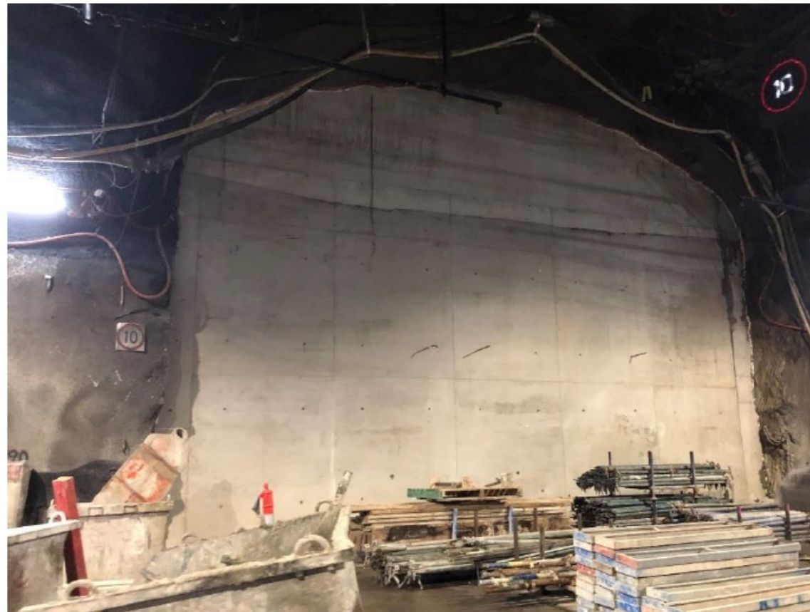
Image 1: PBR final plug complete
