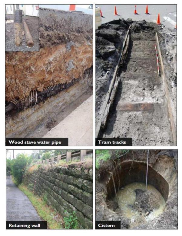
**Top left hand picture continuing clockwise:** Woodstave water pipe with tar and wire sealing (Horsley Drive); Tram tracks (Sydney); Brick lined cistern (Clyde); Retaining wall (Great Western Highway, Leura).
