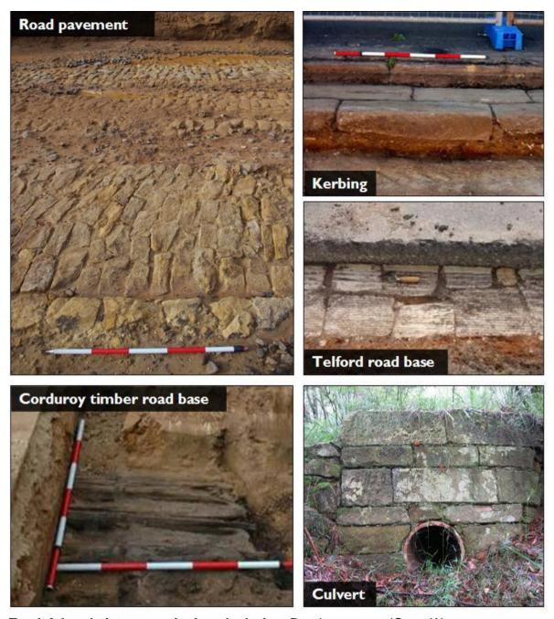
**Top left hand picture continuing clockwise:** Road pavement (Great Western Highway, Lawson); Sandstone kerbing and guttering (Parramatta Road, Mays Hill); Telford road (sandstone road base, Great Western Highway, Leura); Ceramic conduit and sandstone culvert headwall (Blue Mountains, NSW); Corduroy road (timber road base, Entrance Road, Wamberai).
