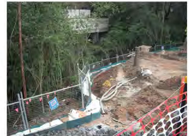
PHOTO 2: MODULAR SEDIMENT TRAP EXAMPLE
