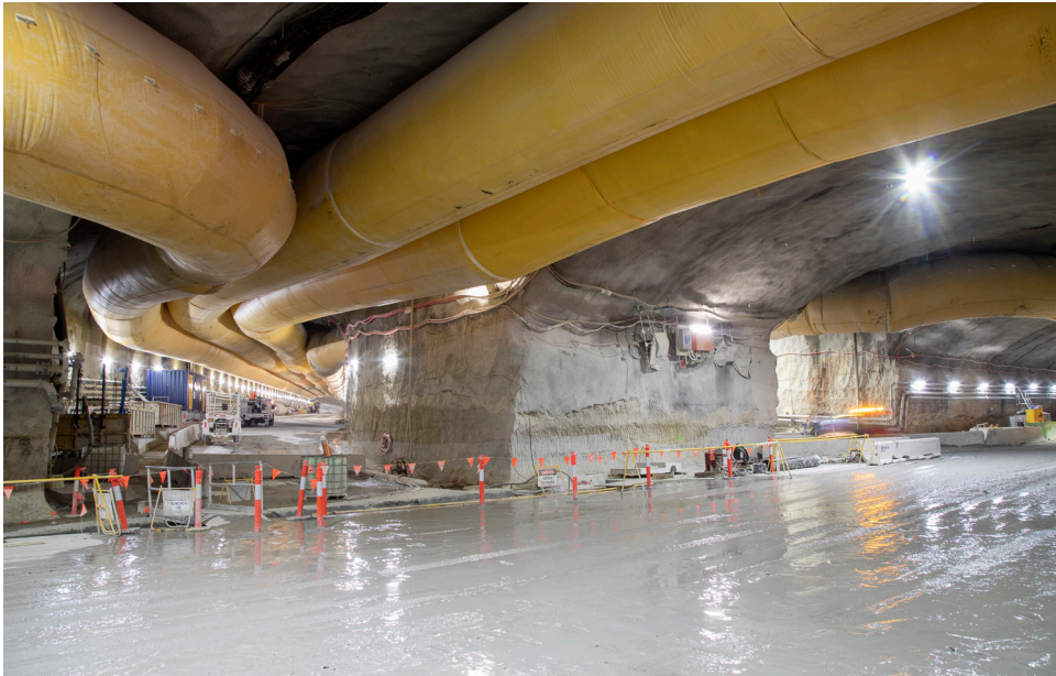
Construction of the M4-M5 Link Tunnels is currently underway
