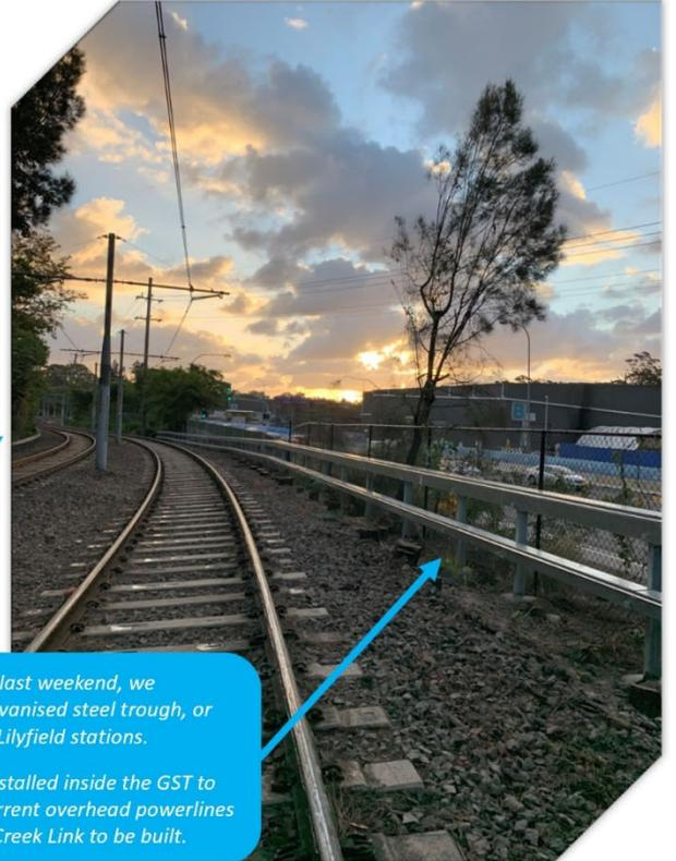
*During the light rail shutdown last weekend, we installed the last section of galvanised steel trough, or GST, between Rozelle Bay and Lilyfield stations.*
