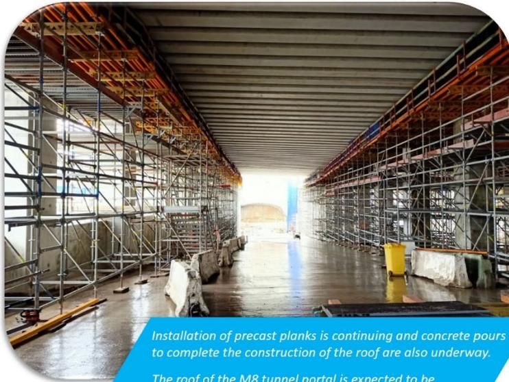
*Installation of precast planks is continuing and concrete pours to complete the construction of the roof are also underway.*
