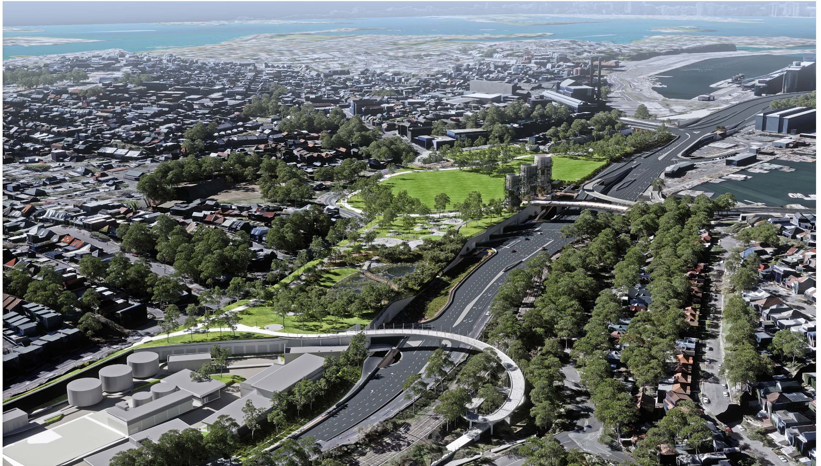
Figure 3: Rozelle Interchange completed project aerial view — artist's impression
