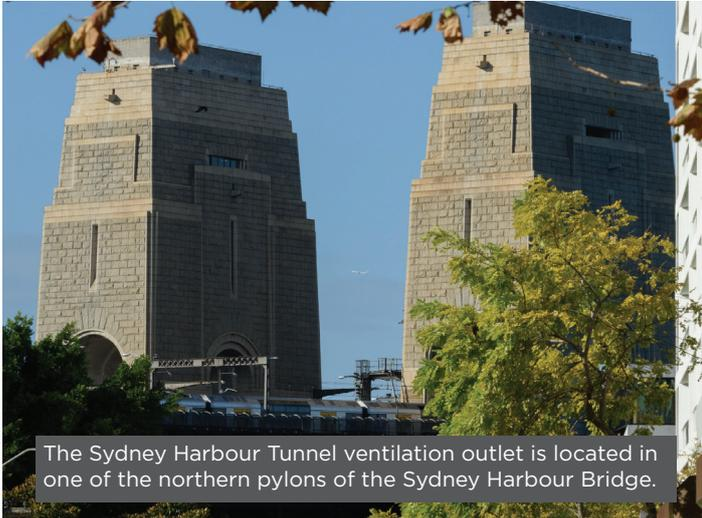
The Sydney Harbour Tunnel ventilation outlet is located in one of the northern pylons of the Sydney Harbour Bridge.
