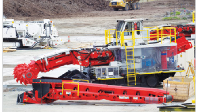
Roadheader at Arncliffe, February 2017
