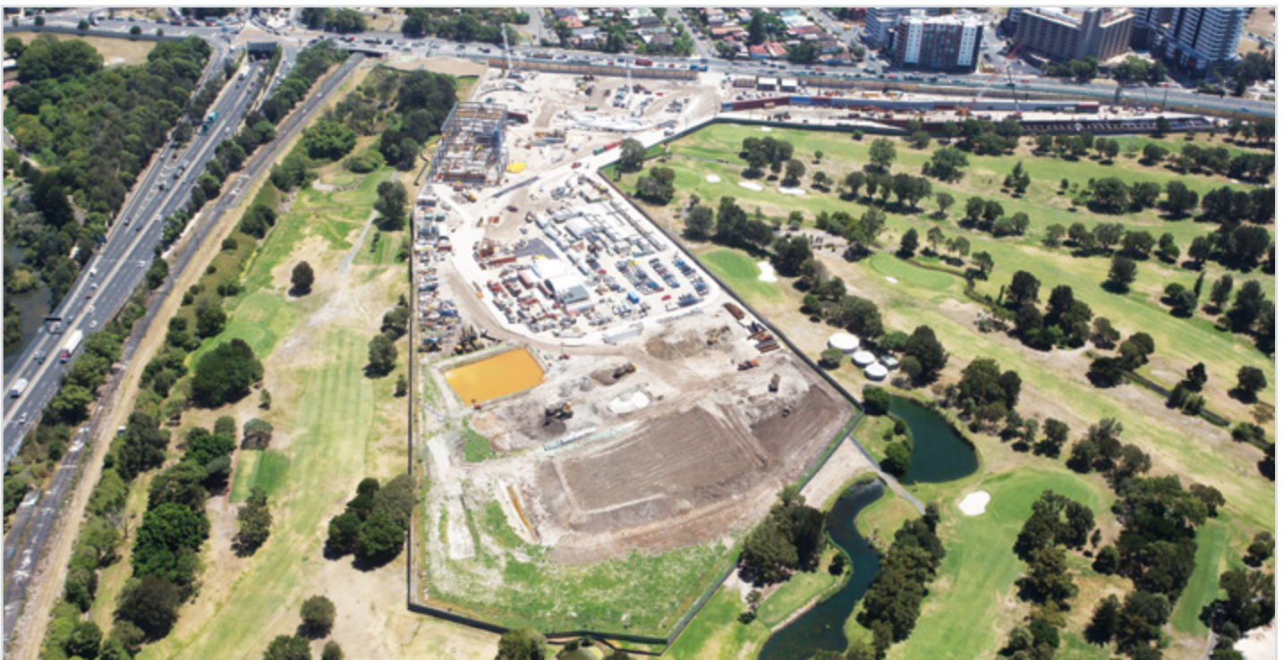
Aerial image of the New M5 Arncliffe site, February 2017
