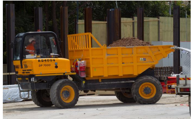
Movement of material on site, October 2016
