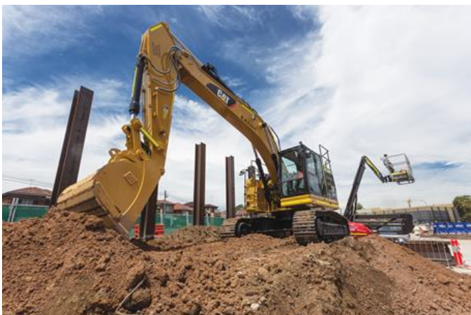
Earthworks at the at the Bexley north site, October 2016
