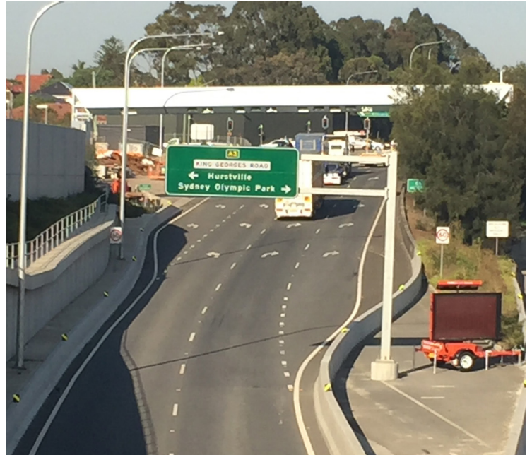
Tolling gantry on King Georges Road
