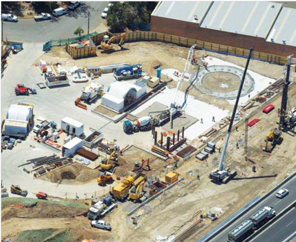
Bored piling to support shaft walls completed at the Kingsgrove tunnel site near Garema Circuit, February 2017
