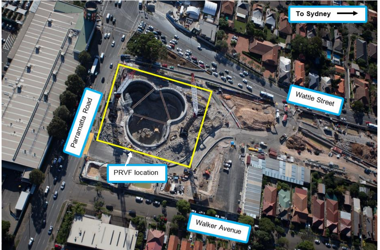
Location of the Parramatta Road Vent Facility, Haberfield.
