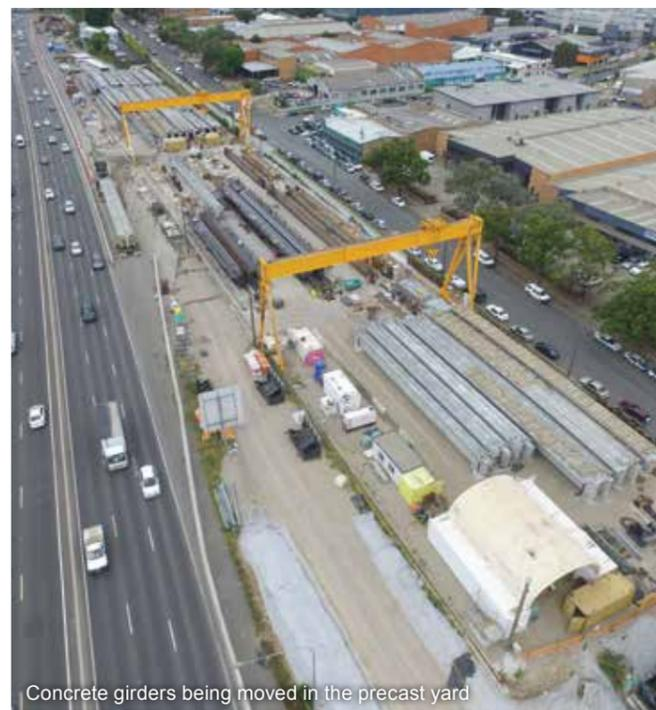
Concrete girders being moved in the precast yard
