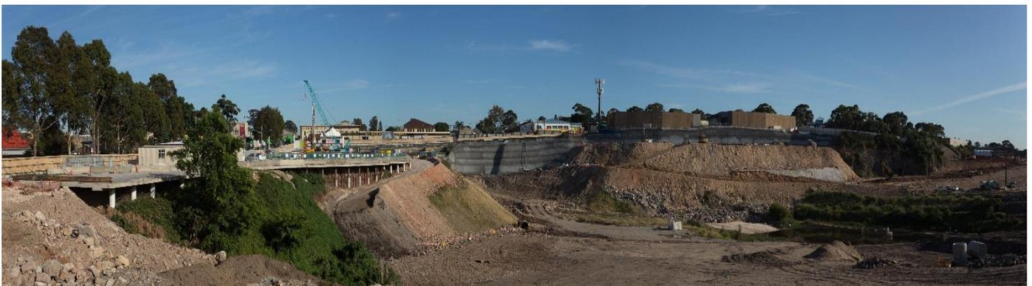
Construction of the tunnel portal, haul road and slope stabilisation at the western corner of the St Peters Interchange site, October 2016
